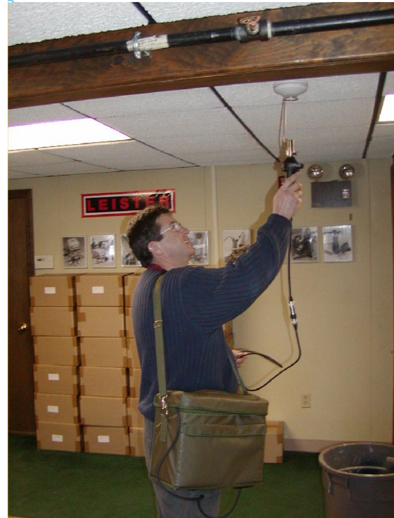
Heat Sensor Testing
