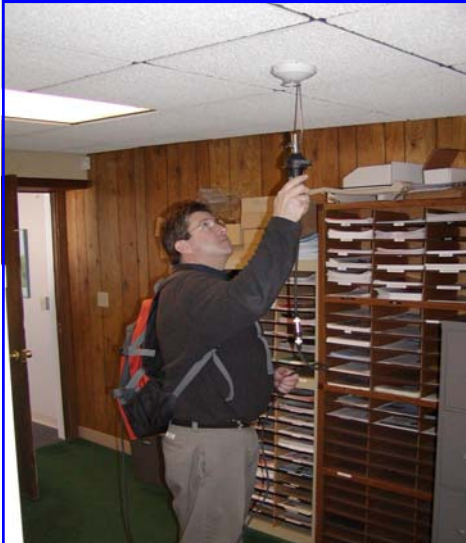
Testing Heat Sensors
