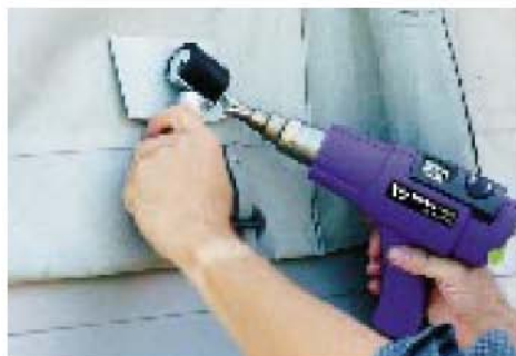
Repair welding on a PVC tarpaulin
