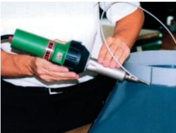
TRIAC PID hand-welding tool with screw-on draw nozzle being used to weld a PVC-U cover.
