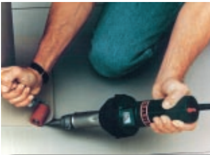
TRIAC PID with 20 mm wide slot nozzle and pressure roller being used to weld TPO roofing membranes.
