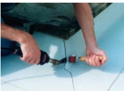
HOT JET S being used to weld PVC-roofing membranes to a skylight. Only 580 g light, the hand-tool is outstanding for welding corners and other detail work.
