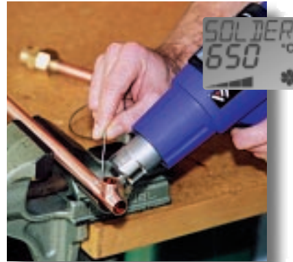
Soldering of copper pipes
