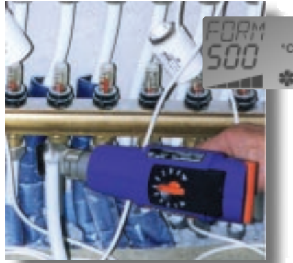
Forming of pipes
